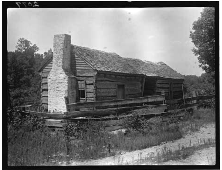
This picture from the Historic American Buildings Survey shows the front detail of an early log cabin near the Meriwether Lewis National Monument in Tennessee. This style of cabin would have been similar to Grinder's Stand, the site of Lewis' death. This was taken by the photographer, A.A. Gustafson in August, 1937. Courtesy of the Library of Congress.
